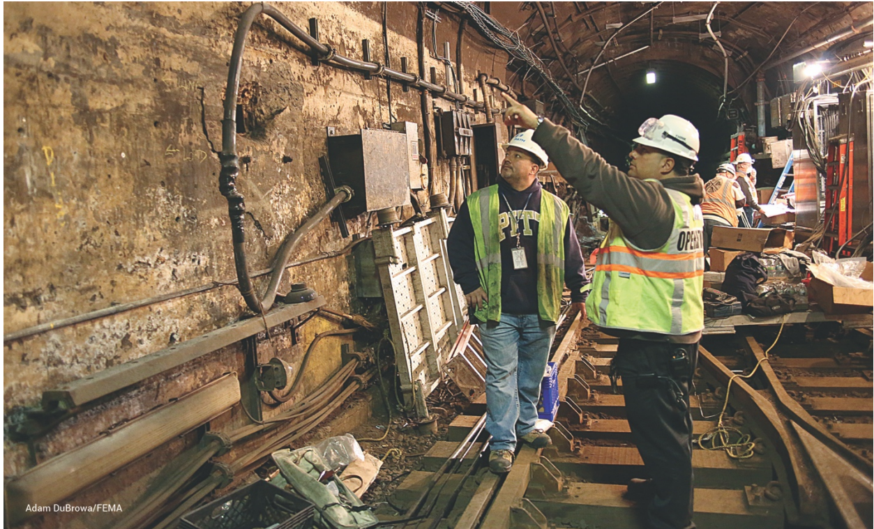
Workers in a PATH tunnel survey damage caused by saltwater inundation during Hurricane Sandy.
