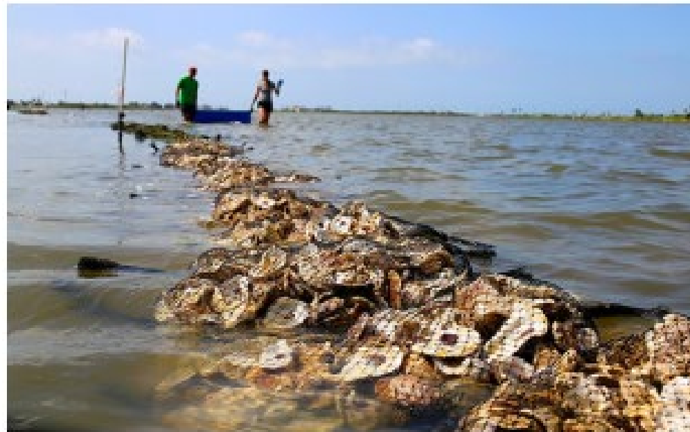
Mesh bags of oyster shells piled to form a breakwater
