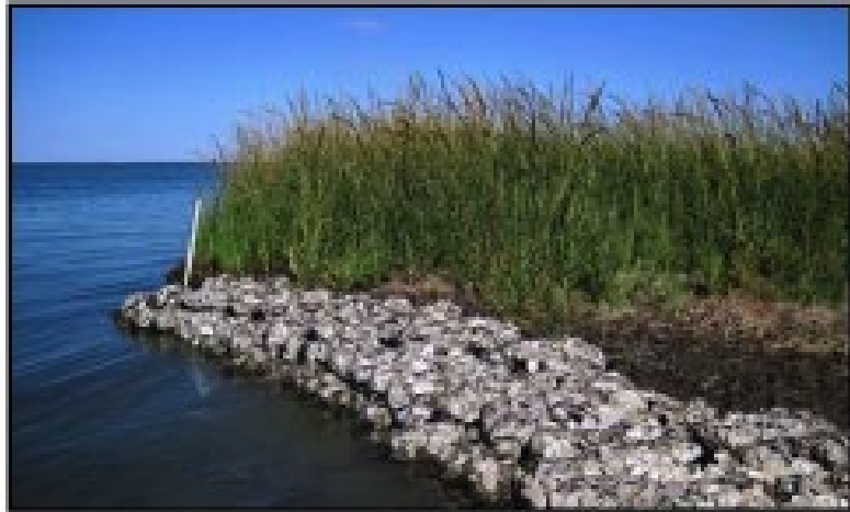
Marsh sills made of oyster shell bag, used with revegetation.
