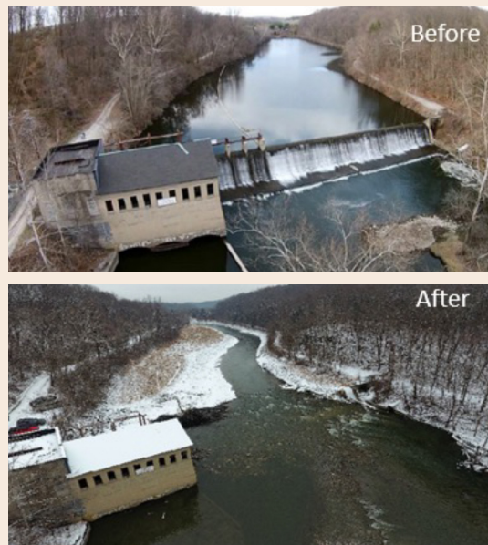
Figure 22. Columbia Lake dam removal before (top) and after (bottom) removal (modified from NJ Dams 2024 ).
